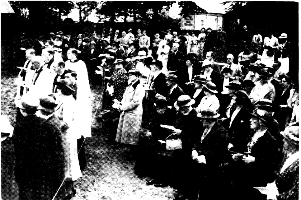
A photograph taken at the Laying of the Foundation Stone of the St. Andrew's Extension on 18th June 1938
